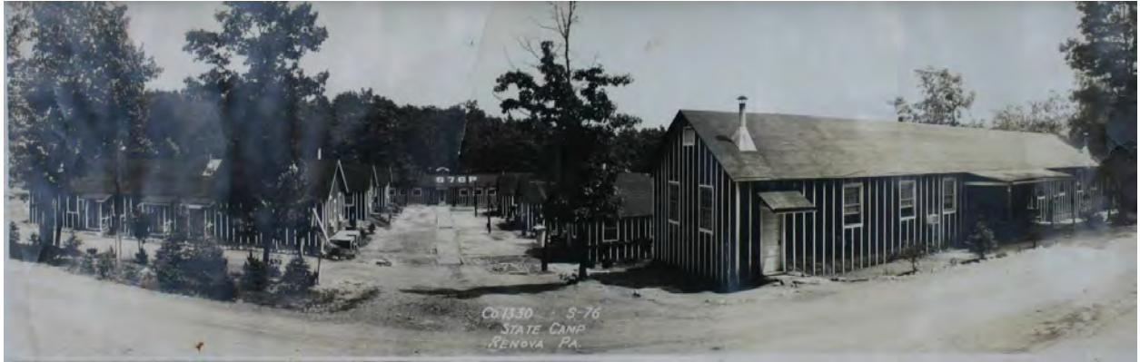
View of camp S-76, Renovo, PA, Company 1330
