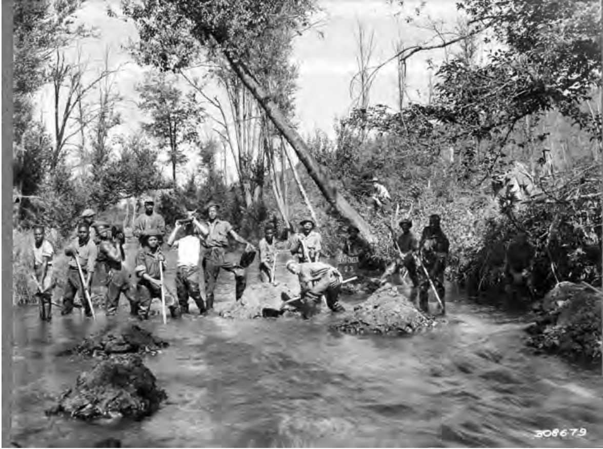
Dam construction at Bear Creek, ANF
