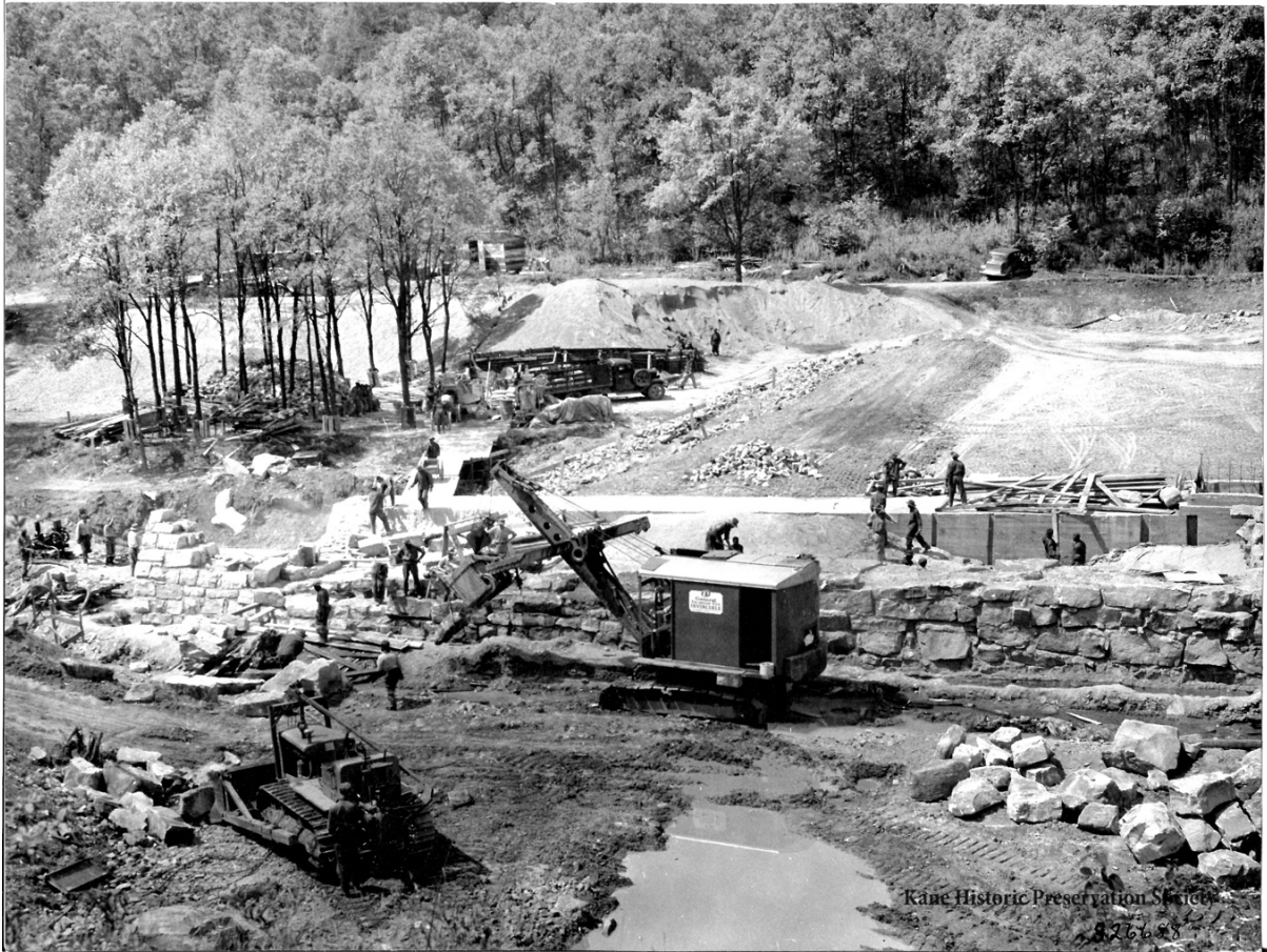
CCC construction work at Twin Lakes Recreational Area, ANF
