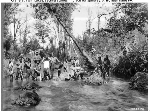
Crane at Twin Lakes, setting stones in place for spillway, ANF, near Kane PA.
