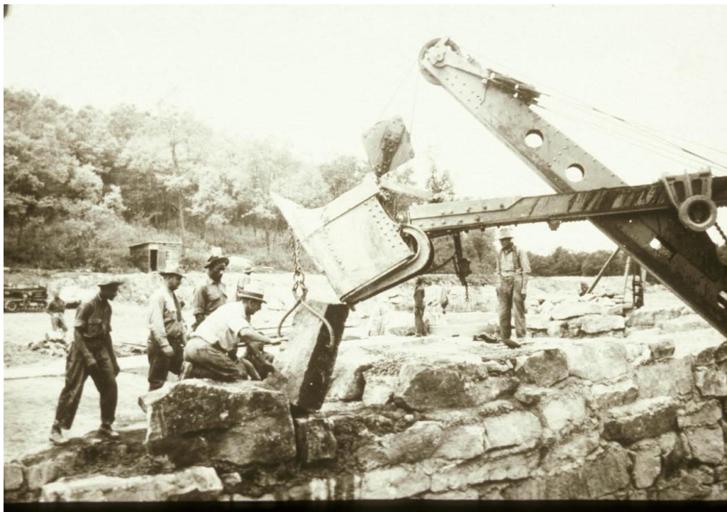
Crane at Twin Lakes, setting stones in place for spillway, ANF, near Kane PA.
