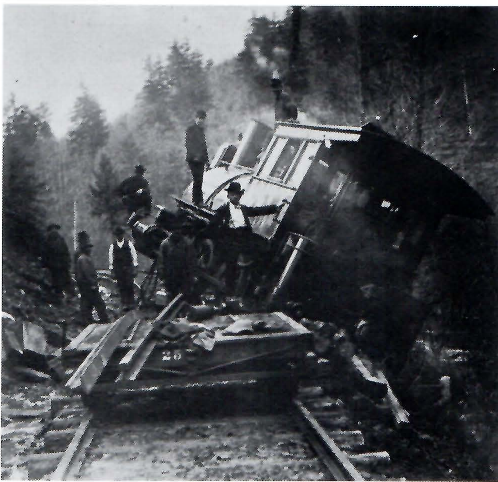
Robert McCullough Cammal and Black Forest R. R. No. 4 jumped the track, narrowly averting rolling down the small embankment. This 0-6-0 saddle tank locomotive was the only rod engine owned by any lumber company on Pine Creek in Lycoming and Tioga Counties.
