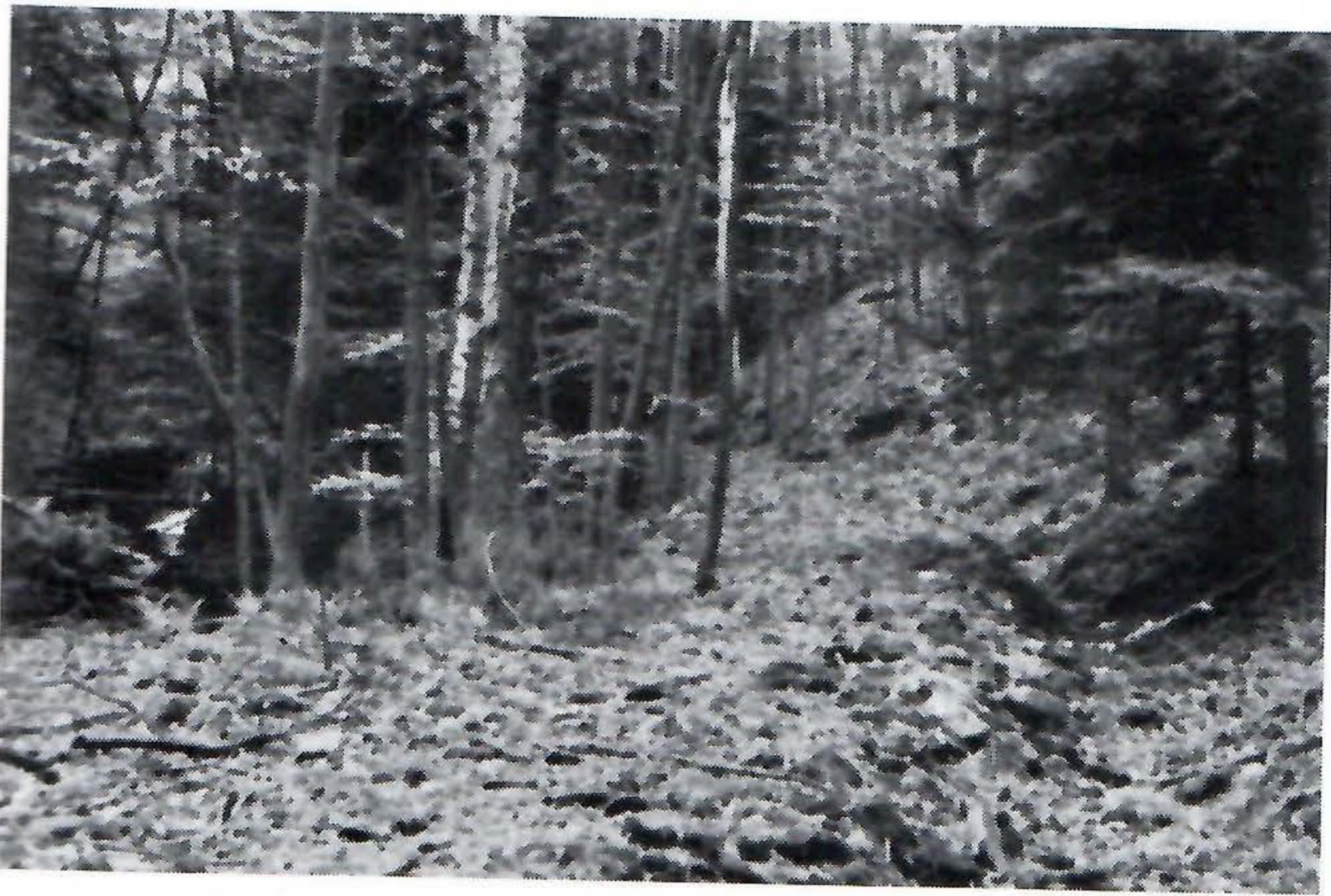
A large curved fill on Sebring Branch that clearly shows the type of grading necessary to maintain a uniform climb.
