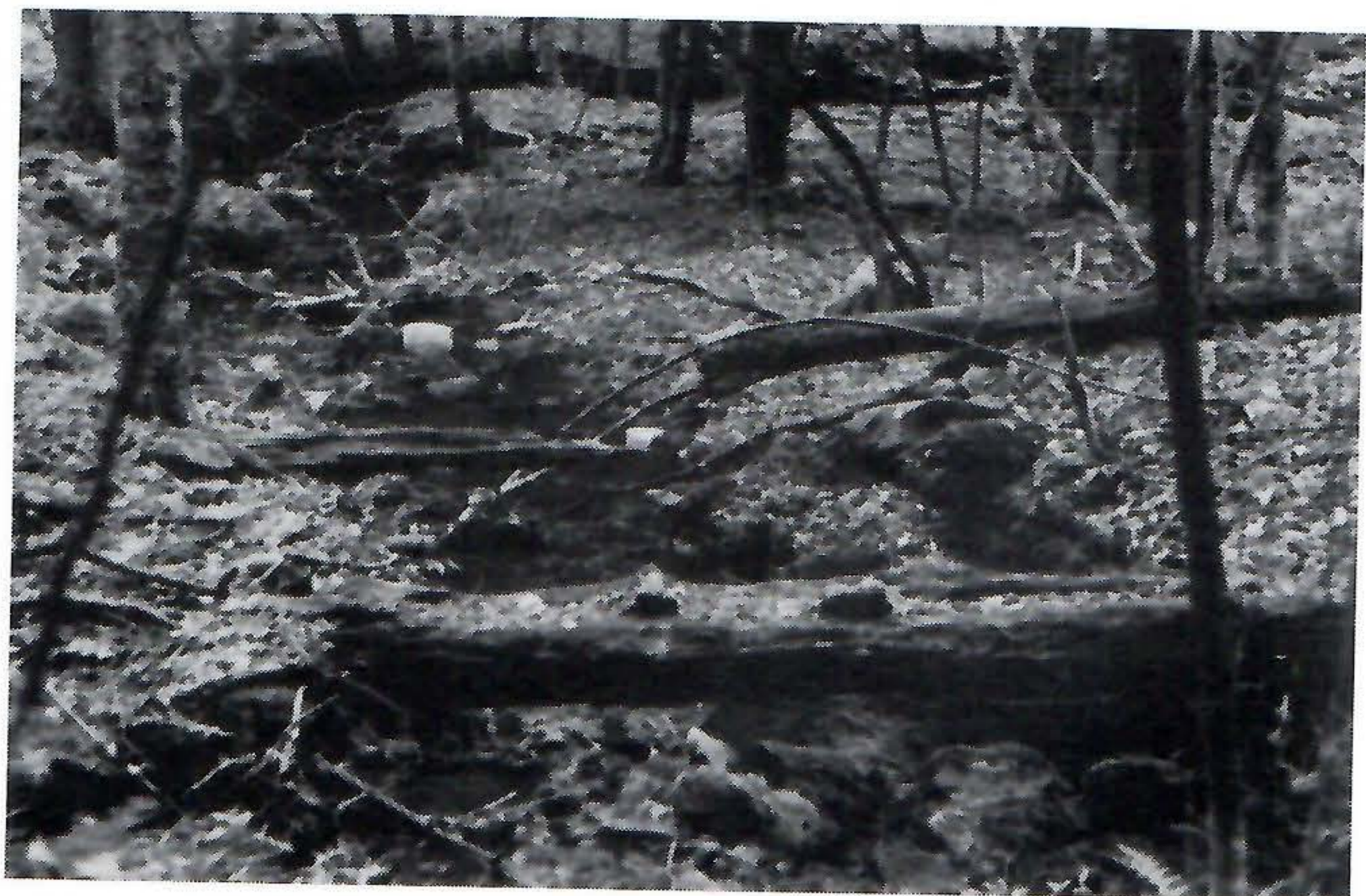
A stringer still remains of the third bridge along the Sebring. Area H of the map.
