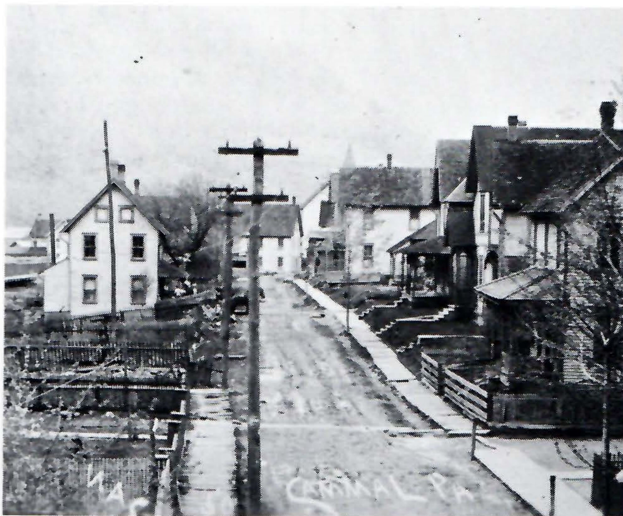
One of the streets in Cammal. Note the electric power lines and poles. A generator at the mill supplied electricity to the village until the mill closed. For the next thirty five years, until 1940, Cammal — and all villages on Pine Creek above Waterville — were without electricity.
