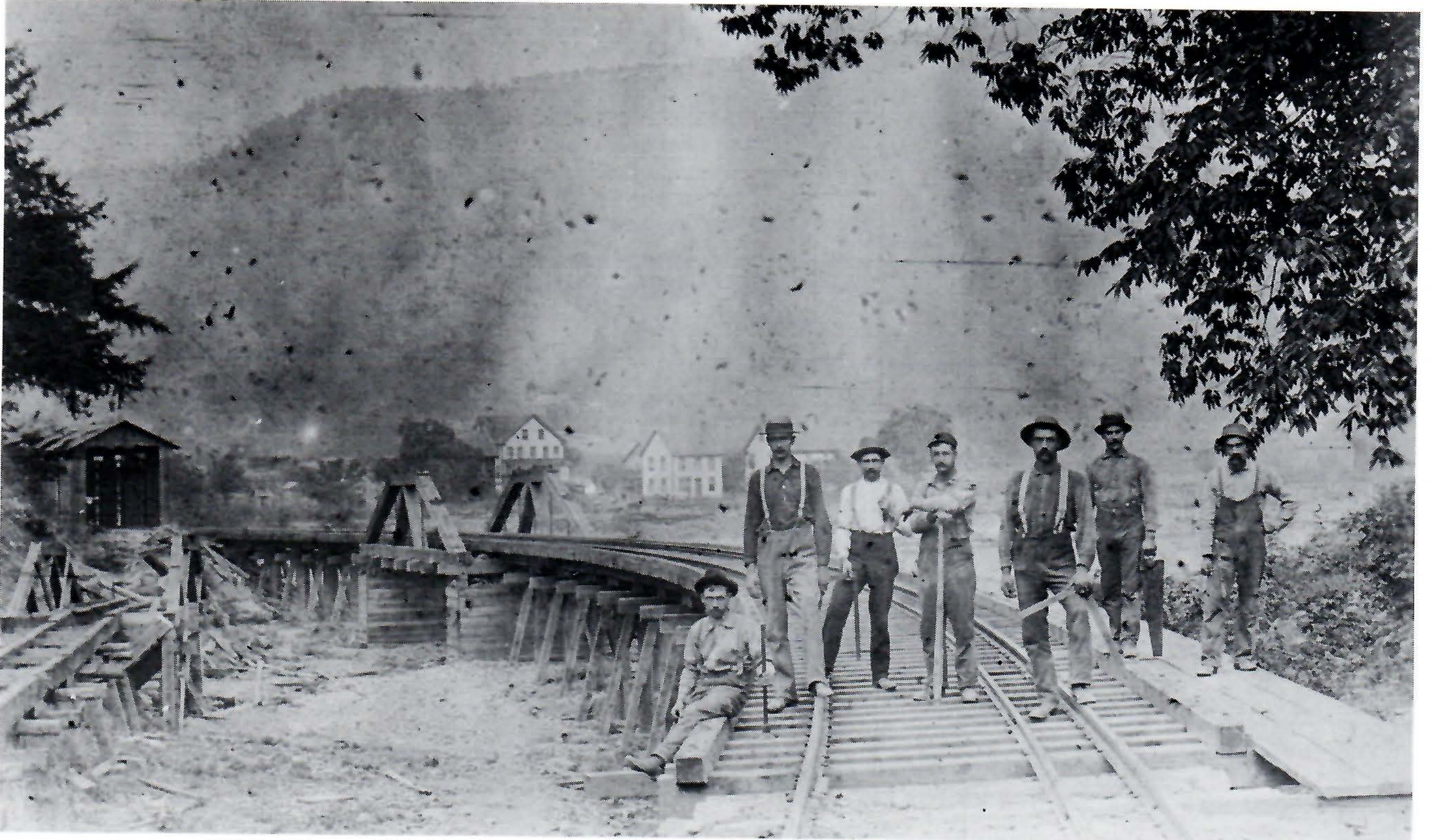
This picture was evidently taken in 1894-95. At the left is the old narrow gauge track leading to the covered bridge over Pine Creek. The new line — narrow gauge for the Trout Run R. R. line up First Big Fork and standard gauge C. & B. F. to Pump Station — had just been completed. Robert McCullough
