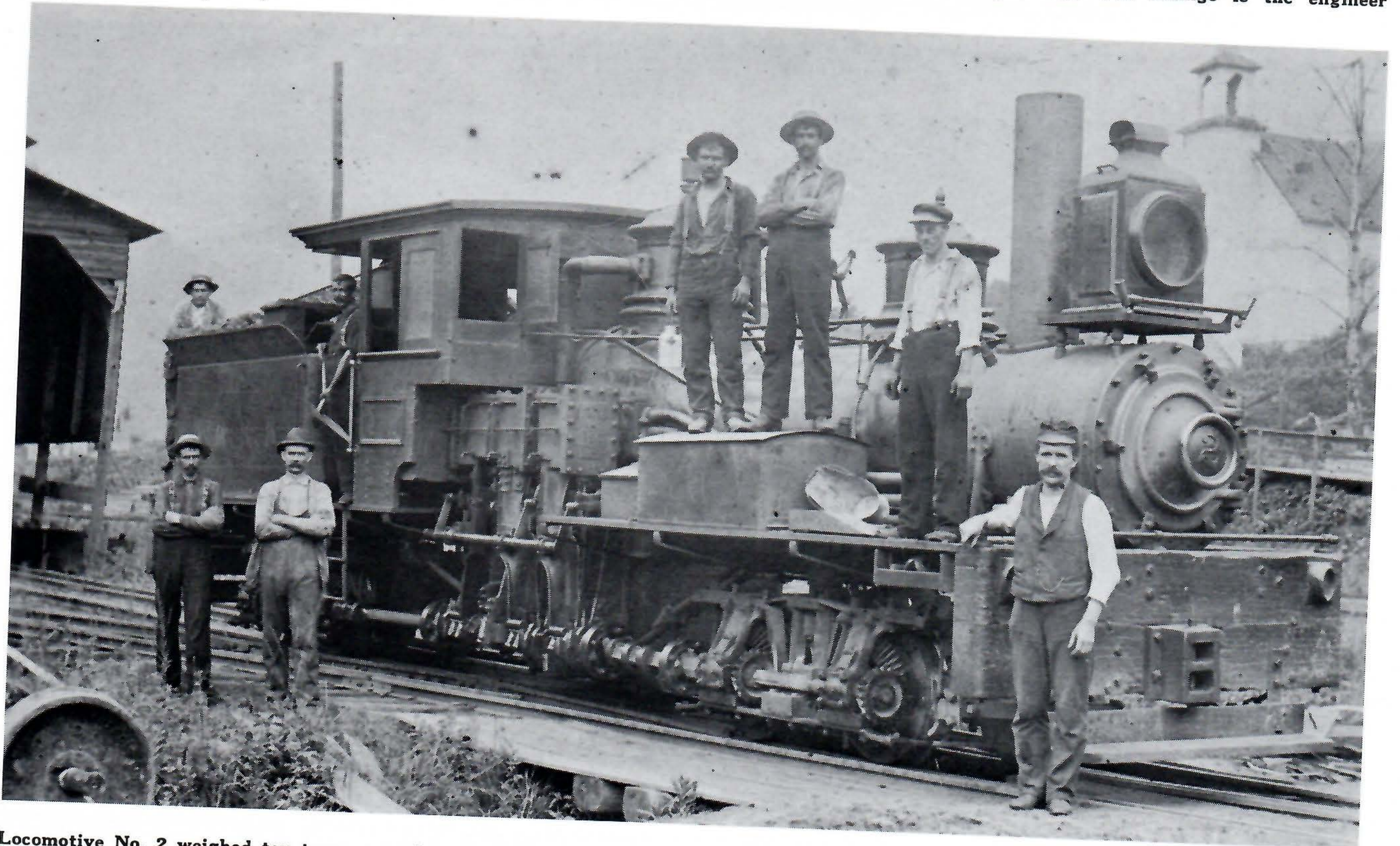
The first locomotive of the Slate Run Railroad brings down a train of standard gauge gondola cars of bark. A narrow gauge log car acts as an intermediate between the link and pin coupler of No. 1 and the knuckle coupler on the gondolas. Pat Iddings is the engineer and Emery Tomb is at the rear of the tender.
