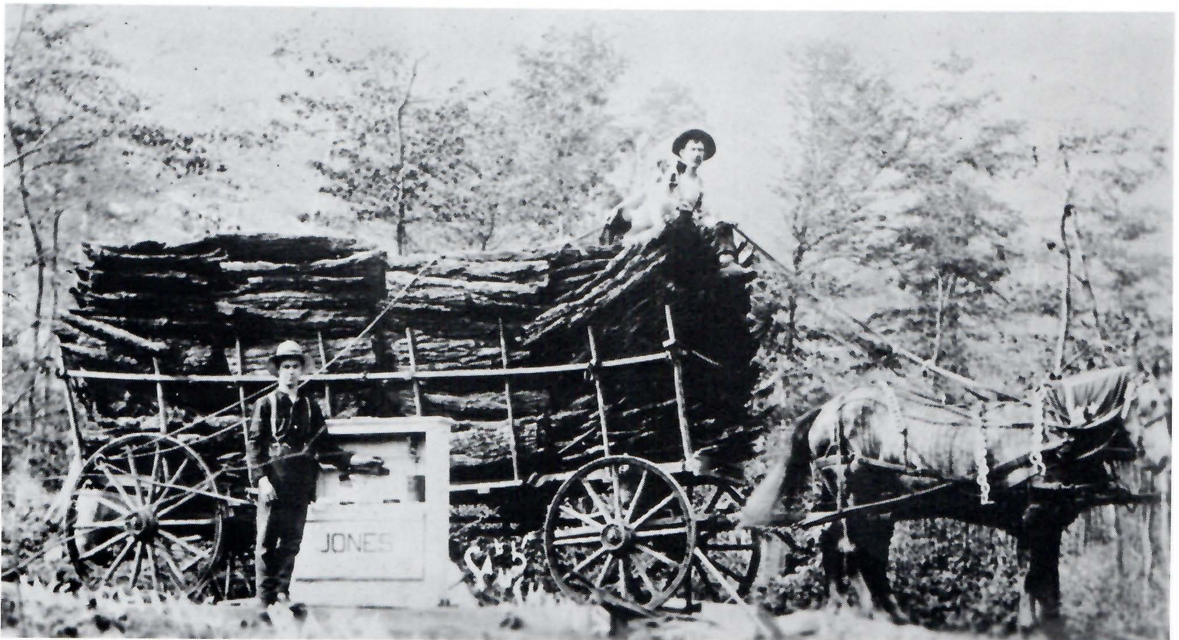
Marshall Welch A load of bark is weighed before being moved to the railroad. Some bark was weighed in the woods, some was weighed on railroad track scales, and probably some wasn't weighed, but was measured. Contracts were to deliver a specific number of cords, not tons.
