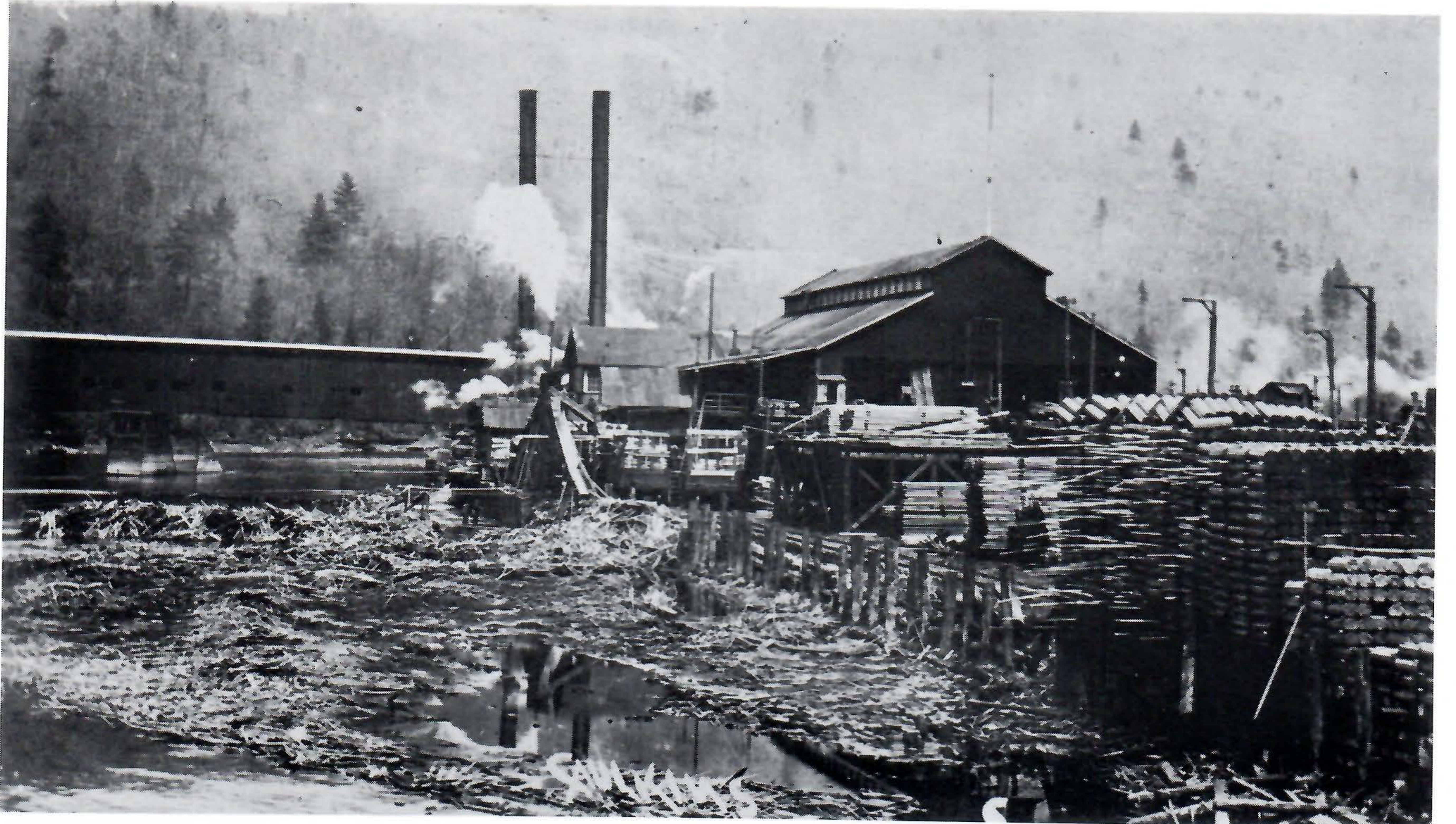
River Pollution! Slab wood waits for high water to wash it down stream. A dam, barely visible, funnelled water thru a flume adjacent to the mill to carry the wood away from the chute. At the right are bundles of lath wood. Back at the mill, beside the slab wood chute, can be seen a gondola freight car being loaded with lath. Marshall Welch
