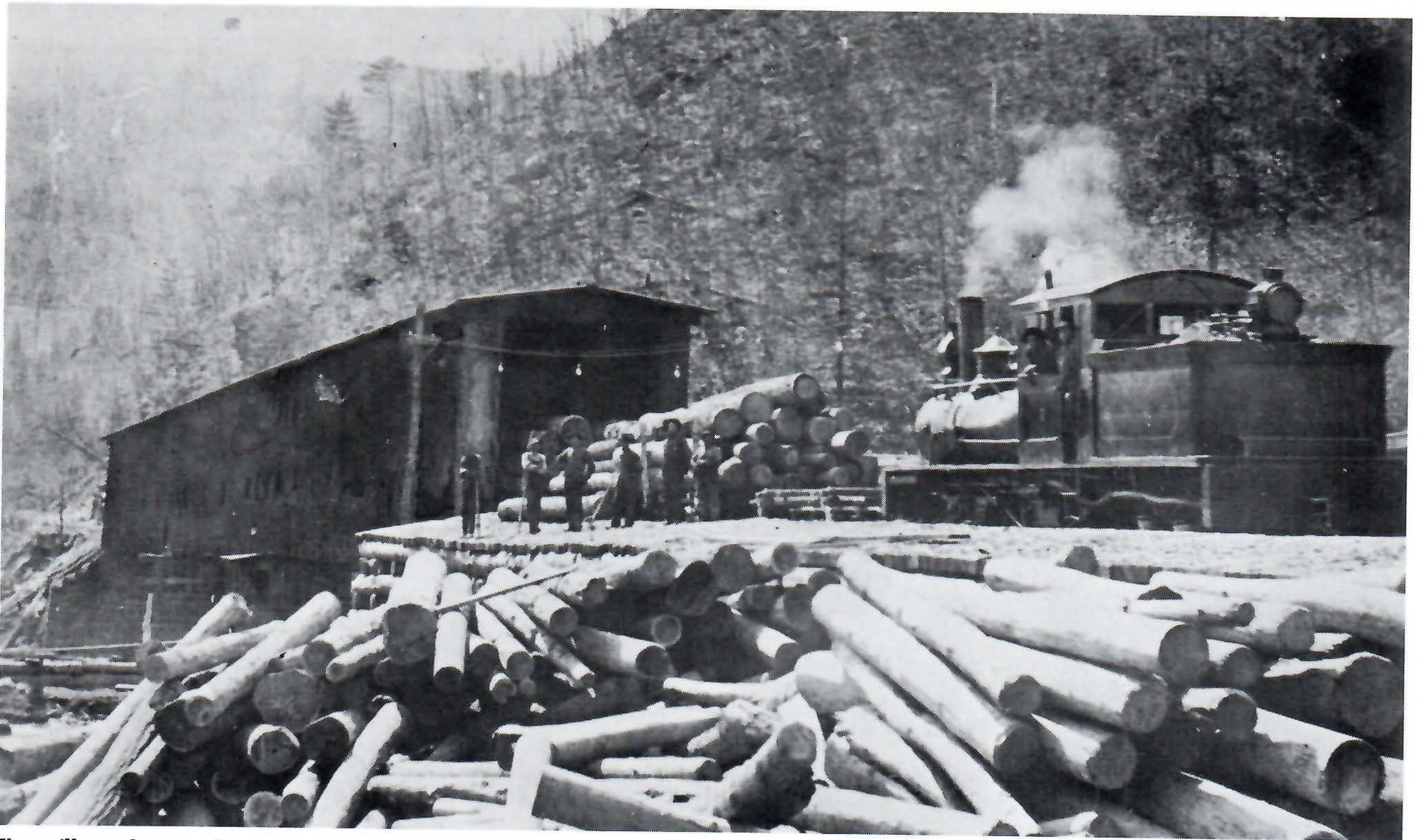
The mill pond was adjacent to Pine Creek. The log train came down Slate Run, circled part way around the face of the mountain, plunged into the covered bridge, and stopped on the other side where the logs were unloaded, two cars at a time. The locomotive is No. 2. The covered bridge had two piers in the creek, and was the longest railroad covered bridge in the state at that time.
