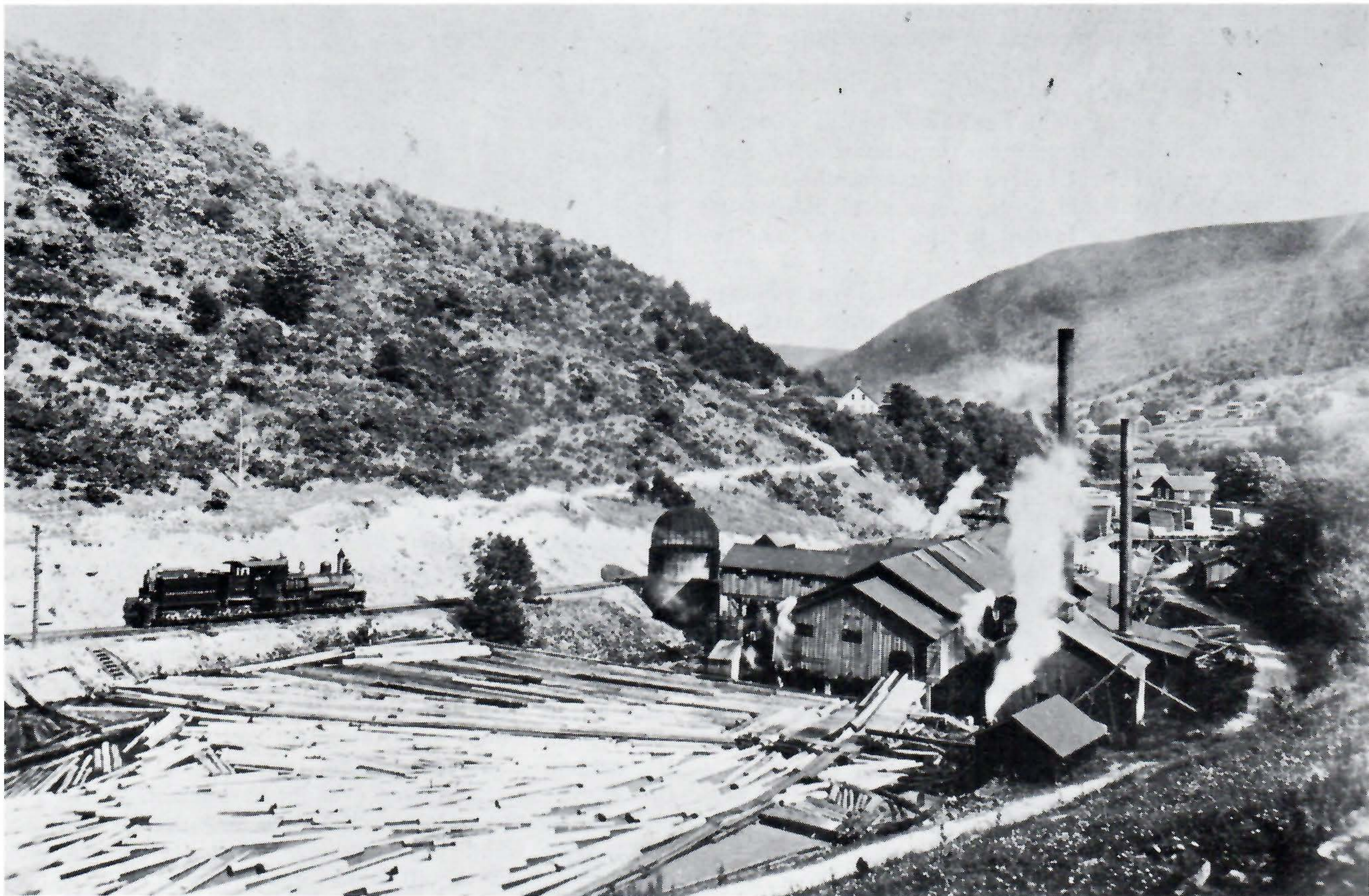
Plamos Louck The mill and pond. There being no kindling wood factory to use the slabs, a wood burner was built to the left of the mill. The locomotive at the pond is No. 202.
