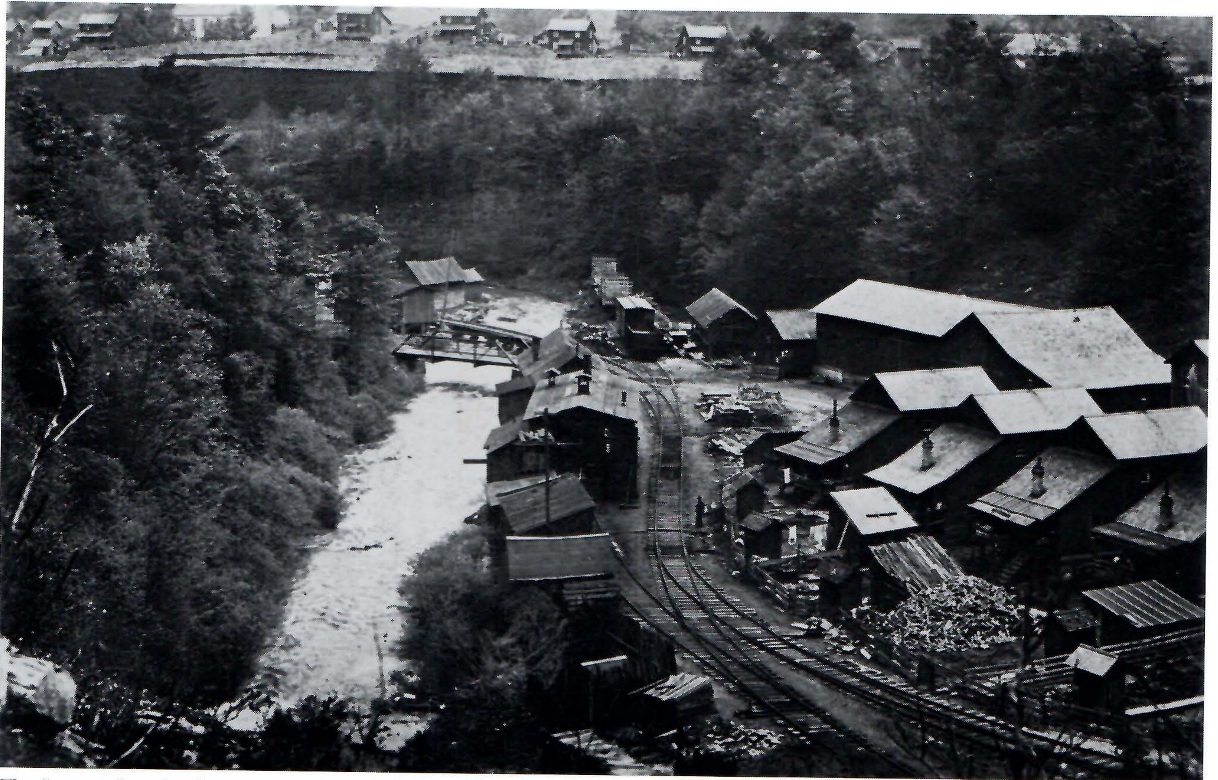
The "narrows" — barely enough room for the engine house, Cedar Run, the main line of the railroad down to the tannery, and the homes of the railroadmen. The house on the right still stands. The frail looking road bridge also remains, and thereby helps a visitor to Leetonia get a proper sense of direction. This view is looking south with the bark stacks in the rear.
