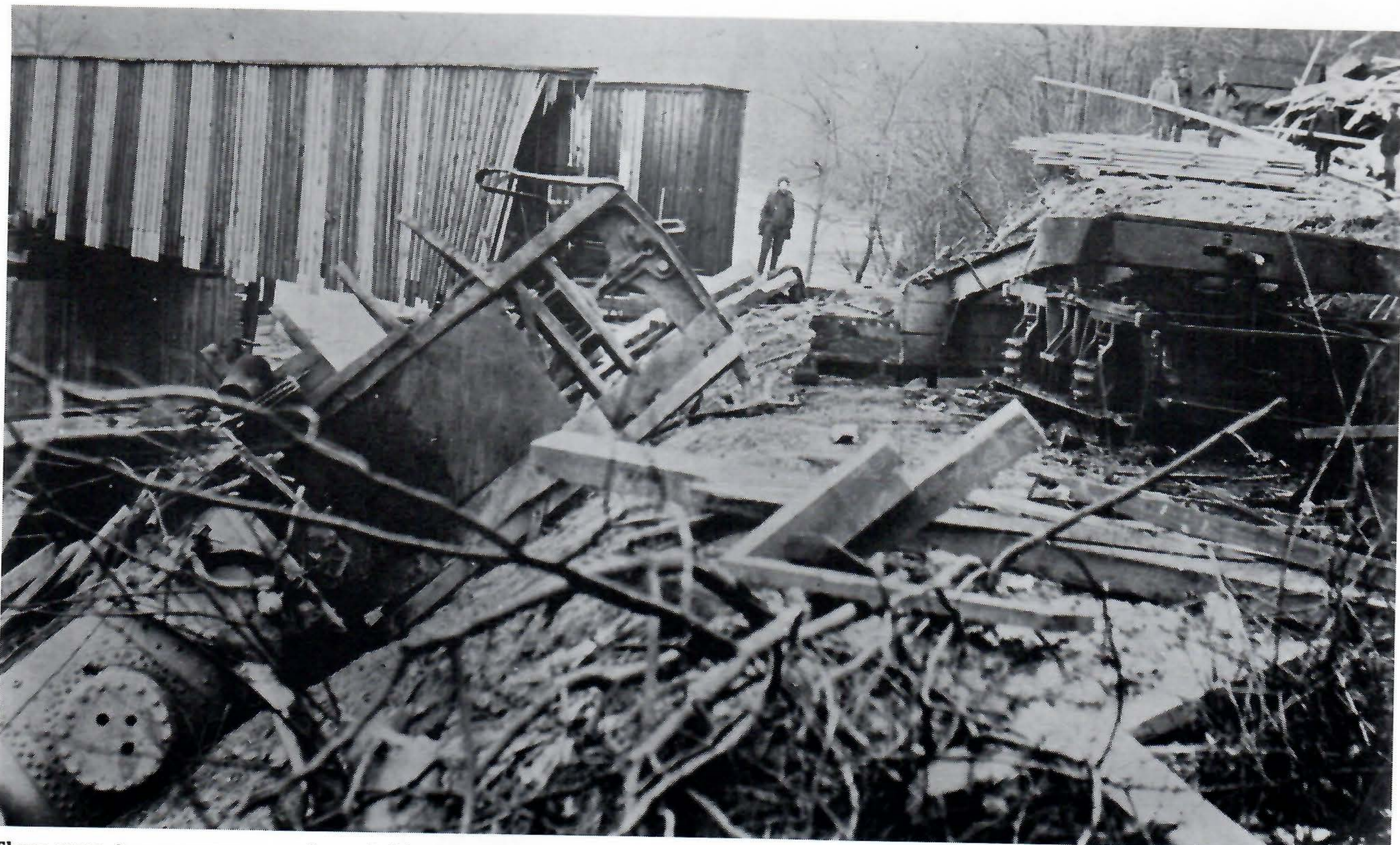
There were two runaways on the switchbacks. Both occurred on the first one as trains were approaching Pine Creek bridge. In September, 1899, locomotive No. 1 was badly damaged. At the time Steven Andrews was engineer; Billy Woodward, the brakeman; and Ed Schobert, the fireman. This picture is the second wreck which occurred on February 13, 1919 with No. 202. Ed Muchler was the engineer. According to Ernest Robinson, a leak in the water tank dripped water onto the sand pipes which then froze shut so that no sand could reach the rail. This, combined with the failure of the brakes on one of the four cars in the train, proved too much loss of braking power, and the train ran away. No one was injured, but it took close to a year before the locomotive was back in service.
