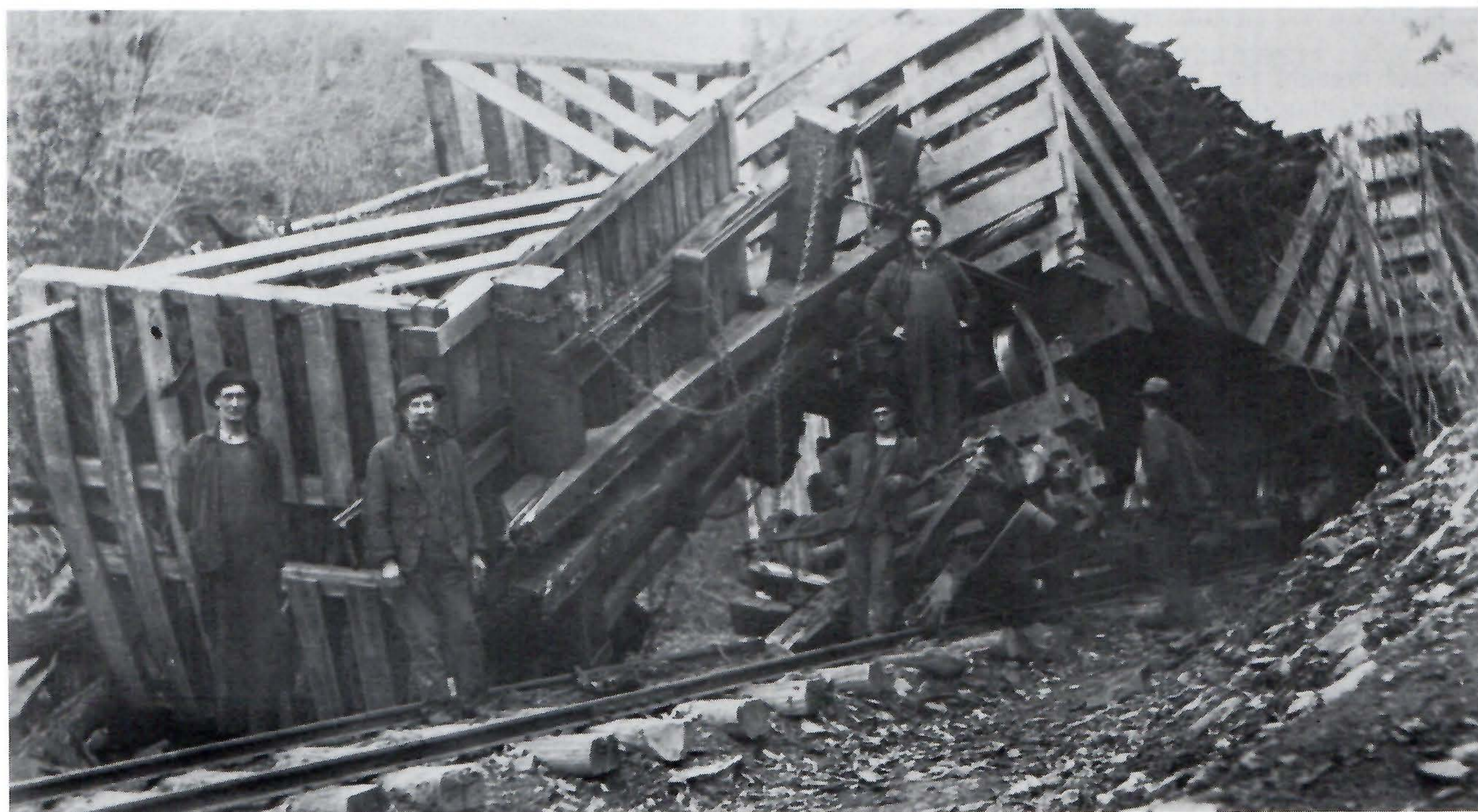
"Tell the carpenter shop we need a few new log cars." A minor accident when a bark car being pushed by the locomotive derailed, and the engine kept pushing.
