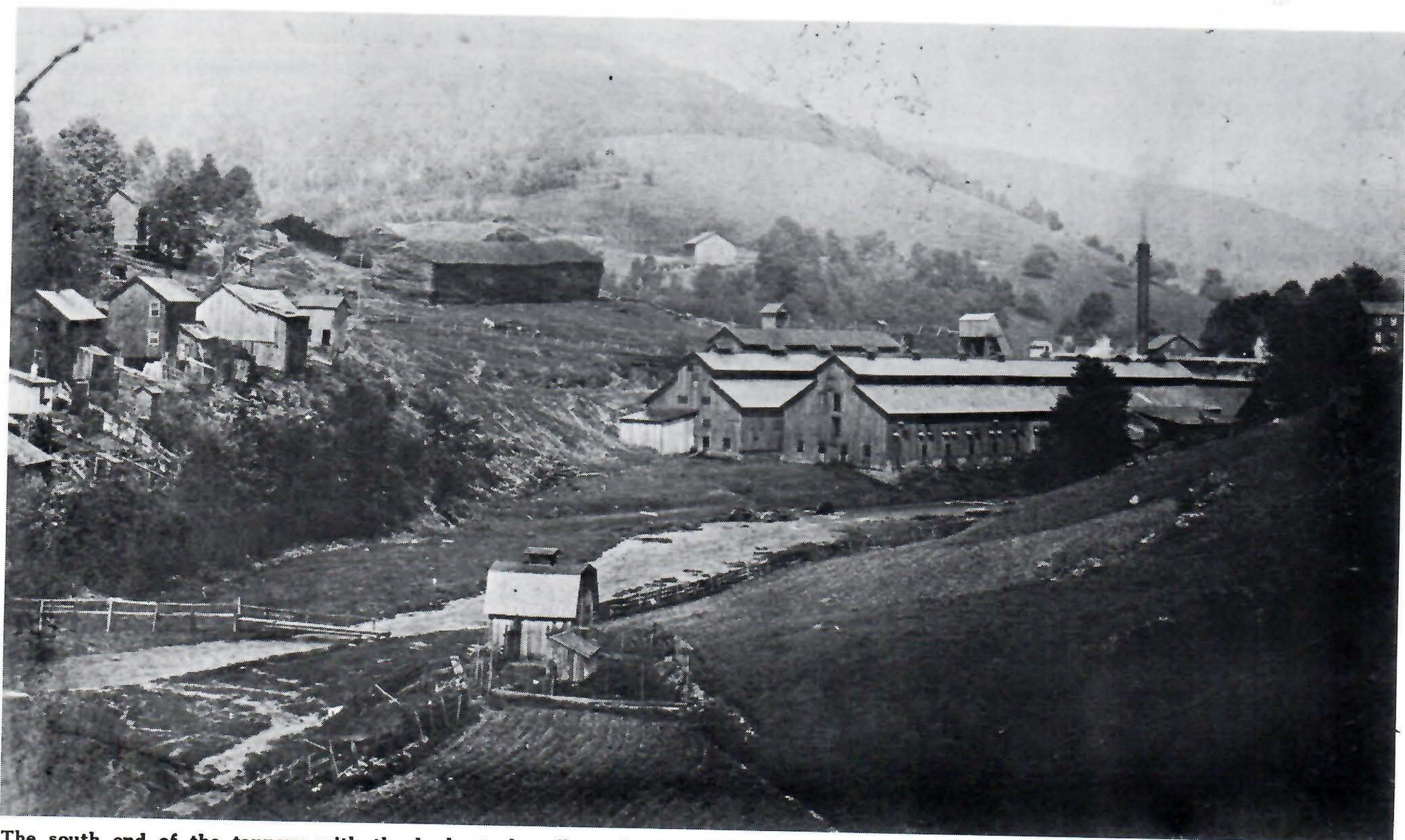
The south end of the tannery with the bark stacks off to the left. Today, the entire area is overgrown, and there are no large open fields.
