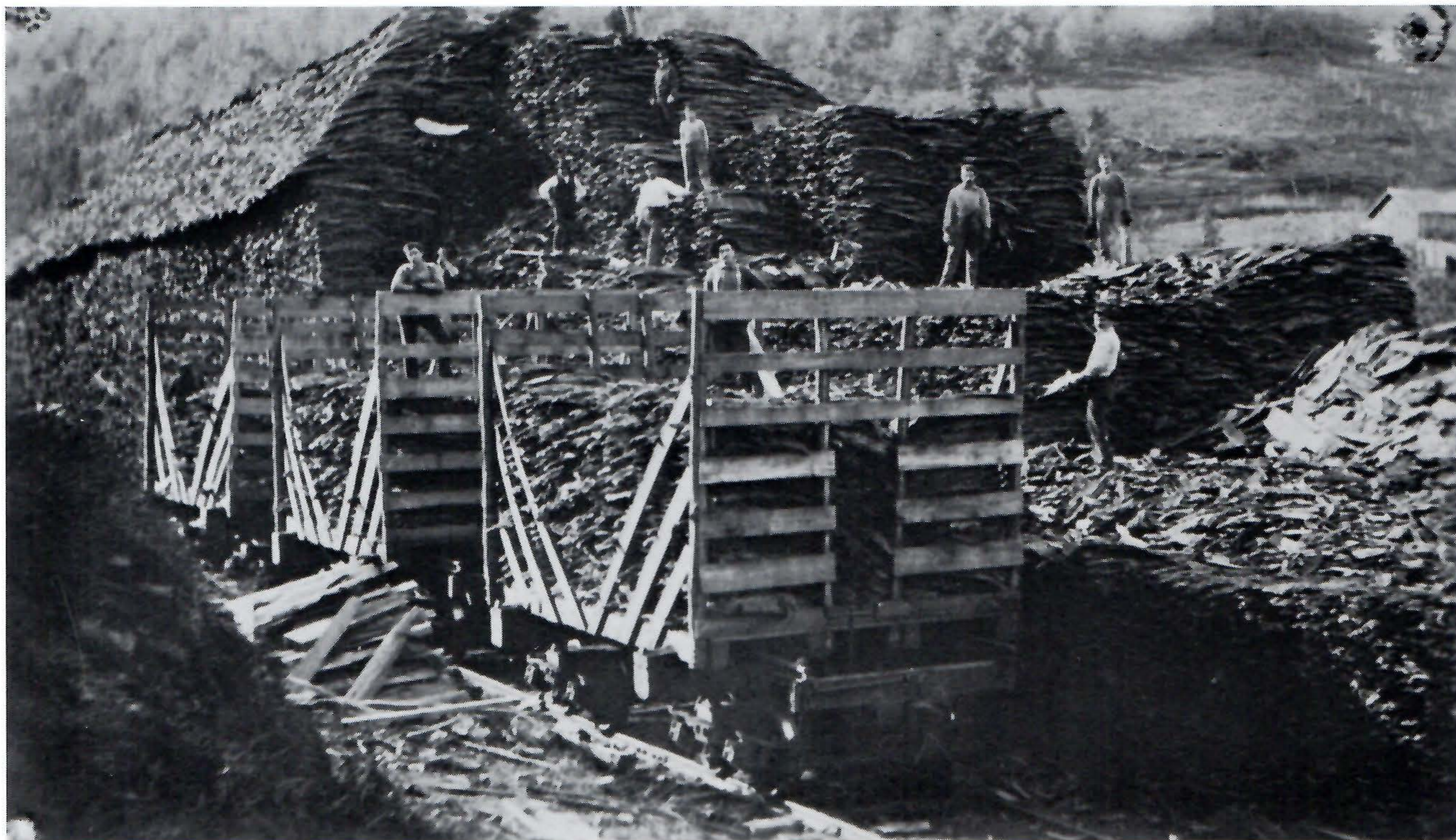
Cars of bark are being unloaded onto the giant bark pile that stretched in front of the school. Because the bark season was only four or five months, log cars were used for hauling the bark. A frame was placed on the car to hold the bark. Ten men appear to be involved with the unloading. Each piece, cut in four foot lengths, was handled individually, being given from one man to the next until it reached its storage place on the pile. Originally the bark was stored under great open sheds; but when these decayed, the bark was stacked with a peak so that water would run off.
