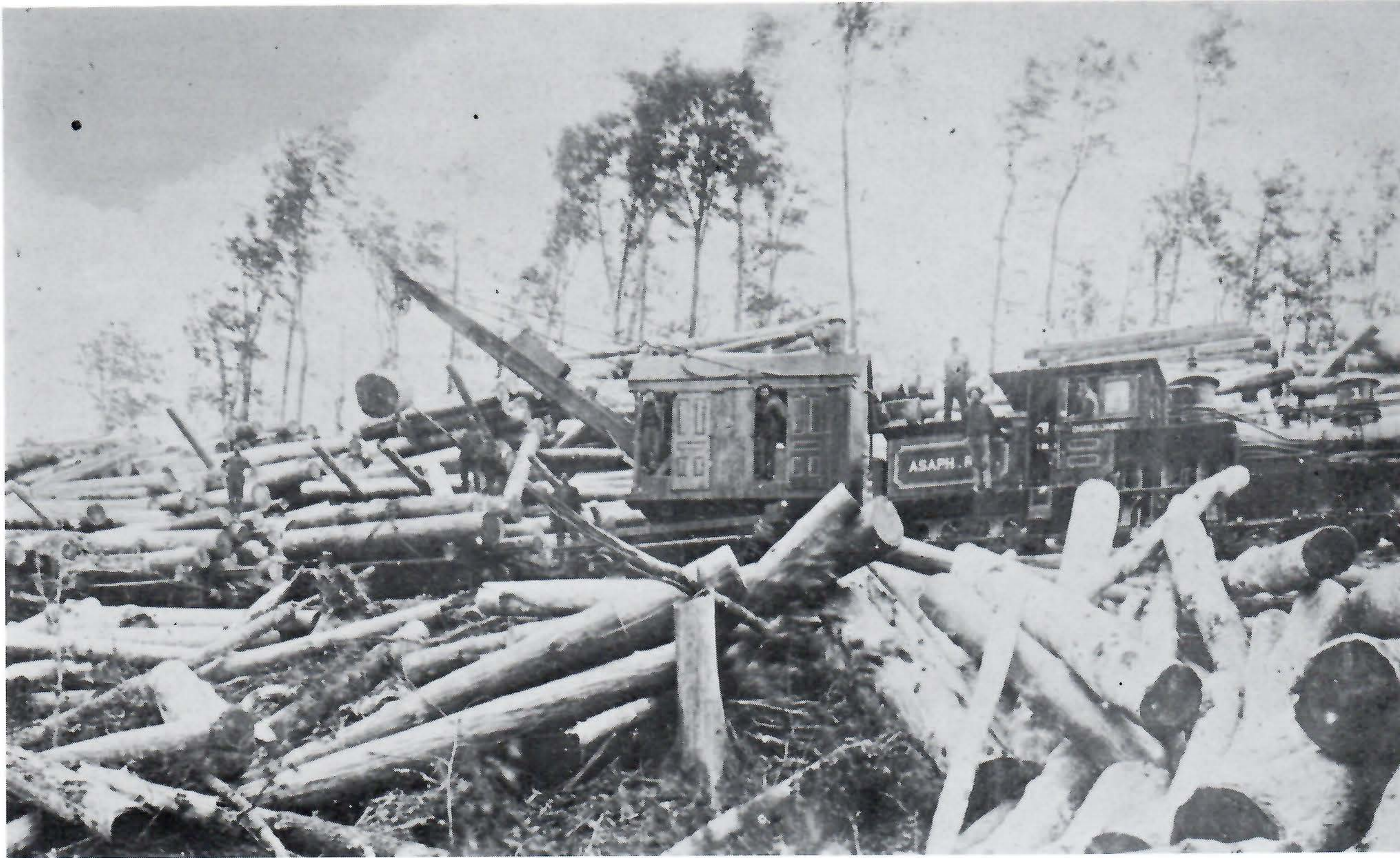
Campbell and Hagenbuch had one Barnhart loader, which was operated by Henry Stricker. Locomotive No. 1, shown with the loader, was an old Shay purchased second hand from an unknown owner.
