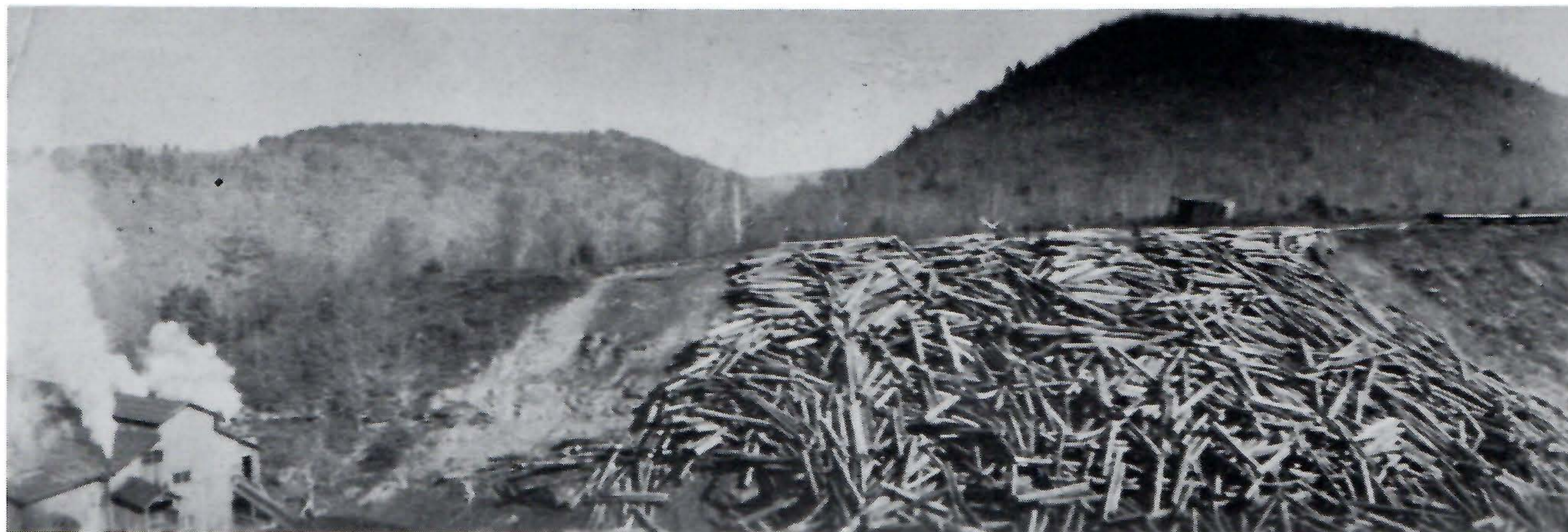
The unloading track of Slaght was on the hillside with the mill at the lower left. The logs were rolled off the cars and down the embankment. Dislodging key logs to allow them to fall into the pond was tricky, but no one was ever seriously injured.
