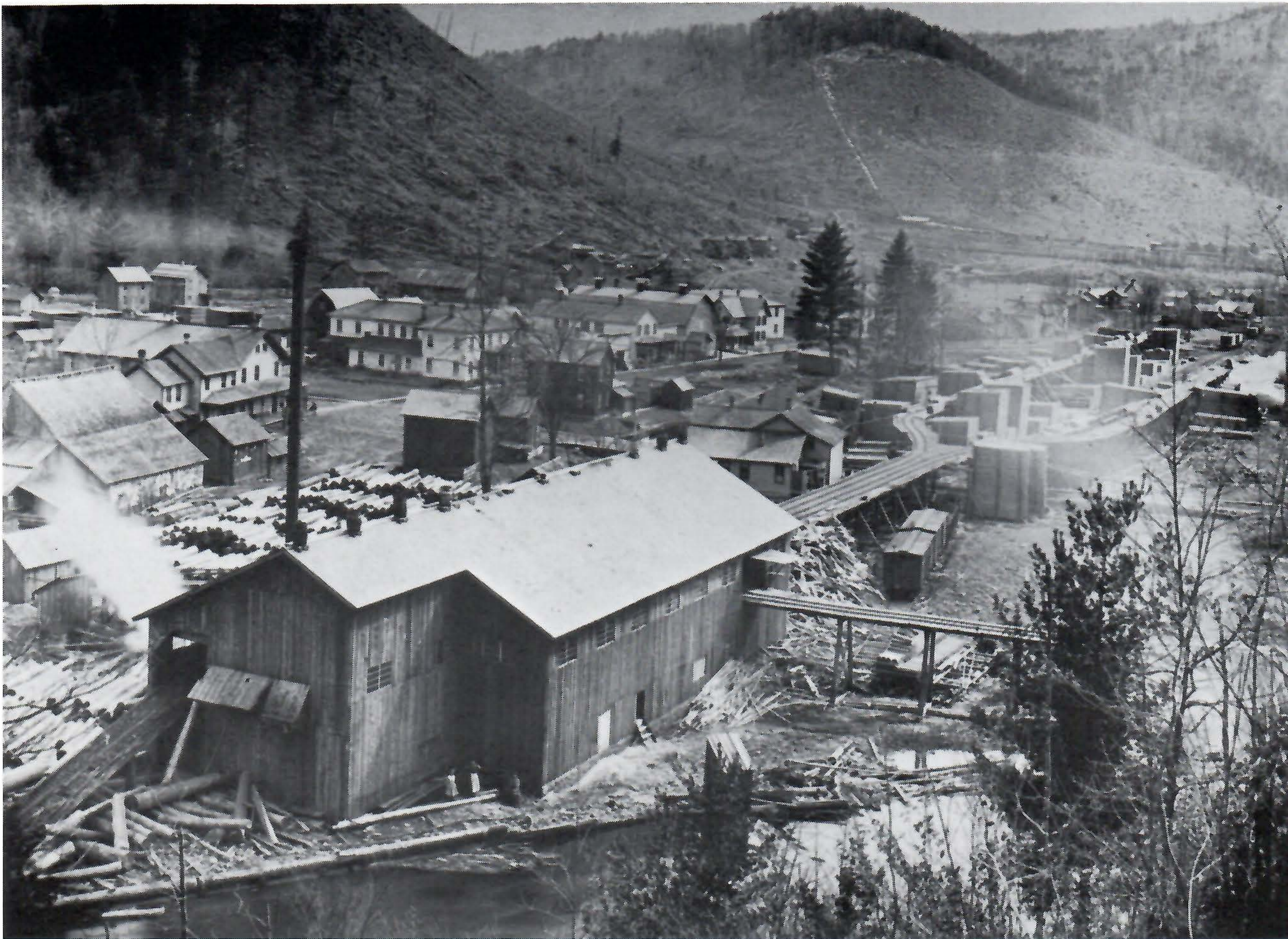
The mill of the Blossburg Coal Company in the nineties. It was situated at the north end of Morris adjacent to Long Run. This view looks south. What is now route 84 passes under the lumber dock just beyond the two box cars. The logging railroad came down from the left, out of view. A few of the homes and buildings in the picture are still standing.
