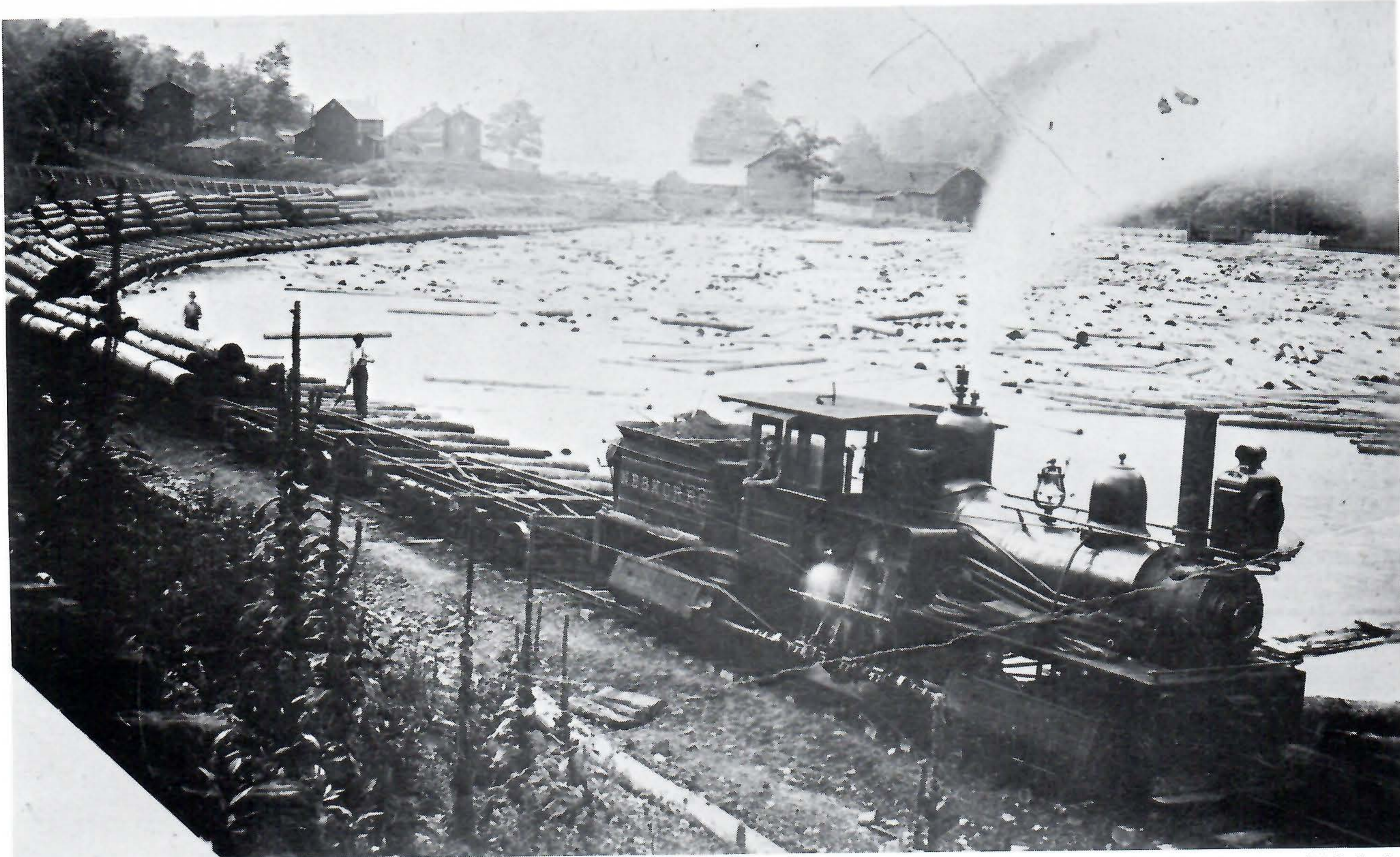
The mill pond for Howard and Perley was huge. A train of twenty four cars could be unloaded at one time. In this picture, which looks south, the first and last two cars have been emptied. At the rear can be seen the pond dam and a bark stack.
