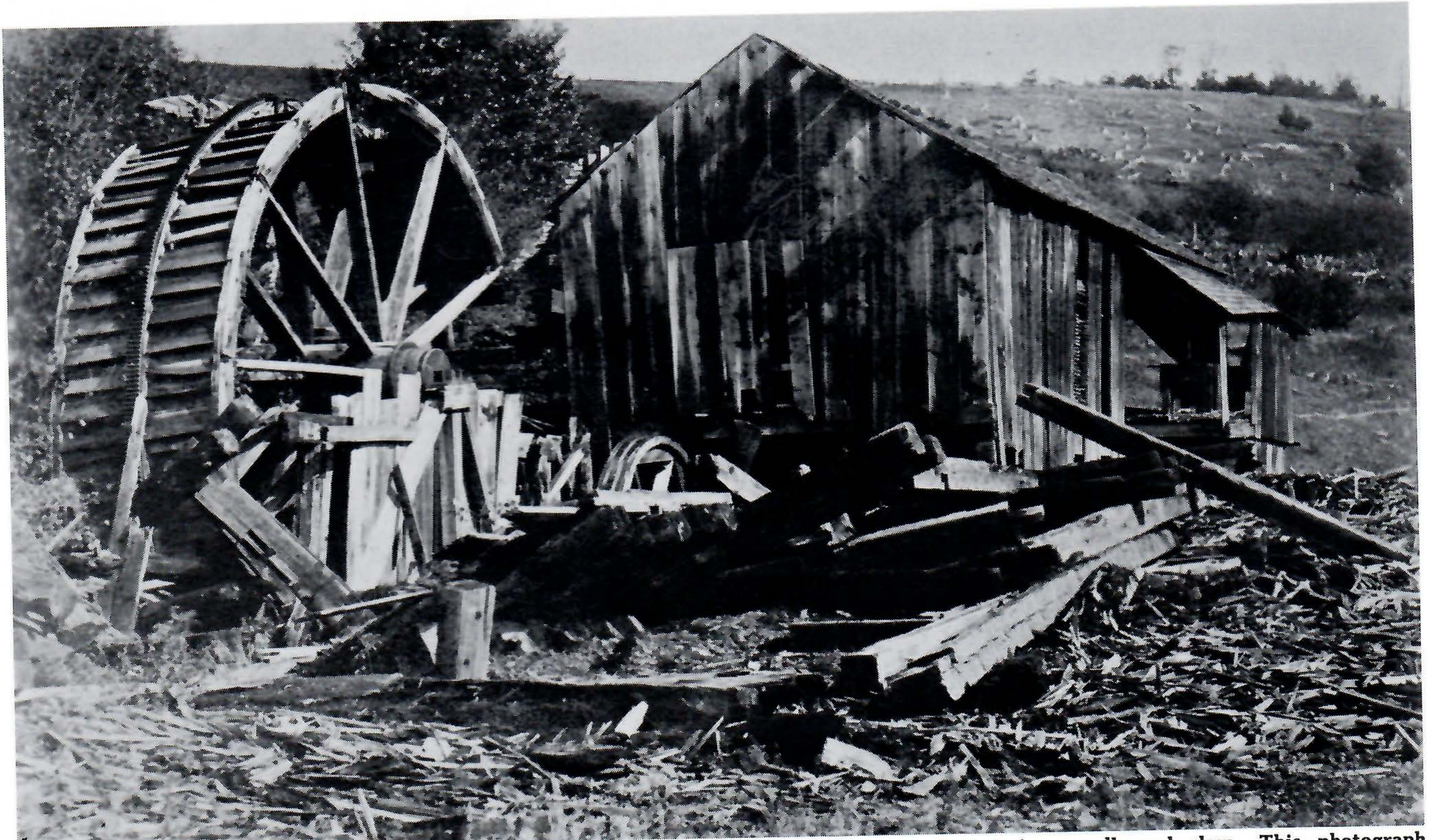
1 The earliest mills in Pennsylvania were water powered. They were usually a family run enterprise, small, and slow. This photograph shows a typical mill. The picture was taken in the 1890s near Hebron, Potter County. Extremely few photographs of water powered mills exist, most having collapsed before photography.
