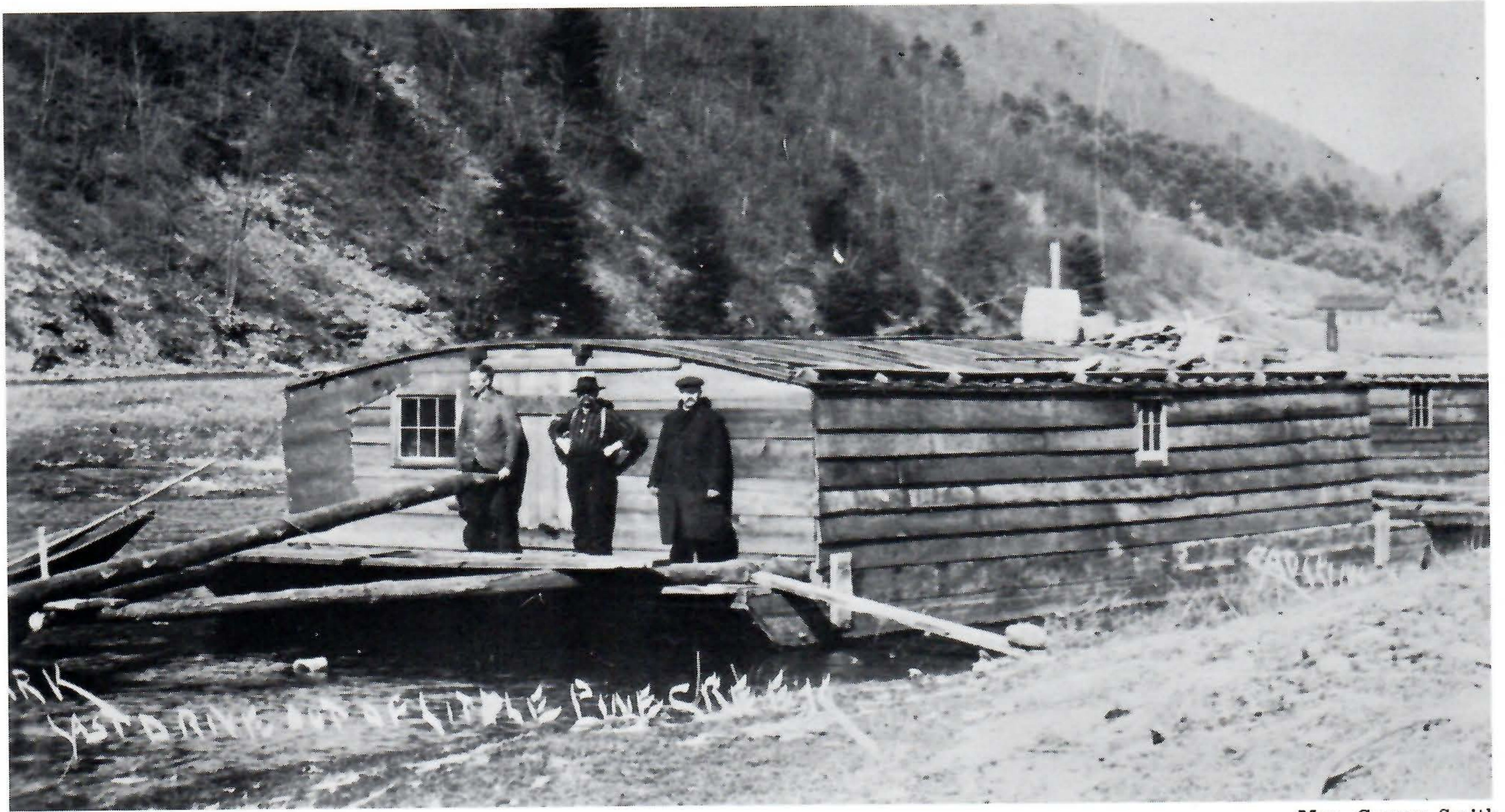
Two of the arks tied up on Little Pine Creek during the last drive in 1909. An ark was used only once, the boat being sold and dismantled after it reached Williamsport. Nelson Caulkins was one of the earliest photographers to photograph "last" events. Mrs. George Smith
